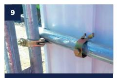
Connect the centre of the first board to the top, middle and bottom horizontal rails, as shown.
