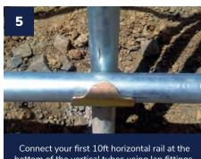
bottom of the vertical tubes using lap fittings, as shown.
