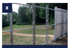
Once the frame work is completed, position the first board at the starting point of the hoarding line.
