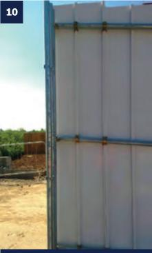
Fit the next board into position and slot into the first board. Connect the board joint to the rails using Go Hoard™ clamps, as shown.
