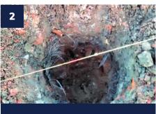
Excavate the holes to the required dimensions (see wind loading calculations).
