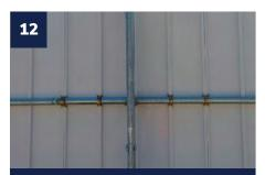
At some points, the board joint may be obscured by the verticle scaffold tube. At these points, the clamps should be fied to the middle channel of the boards either side, as shown.
