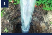
Connect a single 10ft scaffold tube to the 10ft double welded tube, using 3 couplers, and position in the centre of the excavated hole and set in concrete (with plastic sleeves if used).
