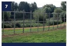
Once the bottom rail is fitted, repeat steps 5 and 6 for the middle and top rails. Placement is to suit your hoarding height.
