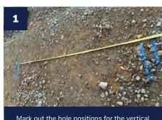
Mark out the hole positions for the vertical scaffoldtubes along your intended hoarding line (see wind loading calculations for spacing).
