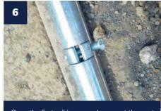
Once the first rail is secured, connect the next rail using a joint pin and secure in place using the lap fittings.
