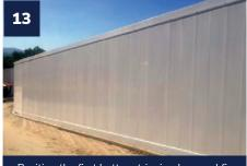
Position the first bottom trim in place and fix using screws and cover caps. Repeat for all top and bottom trims along the entire length of the hoarding.
