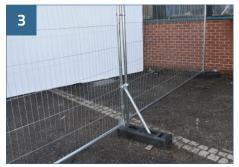
Attach nut and tighten (recommended torque 13NM) to secure brace. Repeat along fence line until installation is complete.
