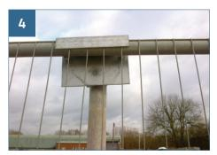
Connect the top BK clamps, as shown, and secure top of the panel by tightening bolts (recommended torque 13NM) ensuring the panel is level.
