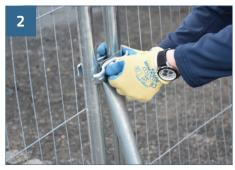
Continue normal installation, placing the panel in front hole. Now remove the nut from one coupler and attach brace as shown.
