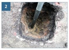
Excavate holes to required dimen-sions and set scaffold tubes in place using concrete (ensure tubes are upright and level).
