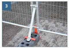
Repeat steps 1 and 2 along the intended fence line and continue as per standard installation, with panels now inserted into ZT base. Ensure the bottom coupler is connected through the anti lift bar of the base, and connect mini brace in the same way as other braces. Ensure nuts are tightened to 13NM.
