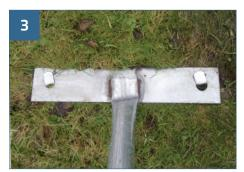
Insert support brace pegs through holes in base plate using appropriate tool, and repeat steps 1 to 3 along the fence line (please note that you should scan for services where pegs are to be placed).
