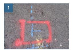
Mark the positions of the holes for the scaffold tubes at the required distance apart along your intended fence line (use 2 scaffold tubes for the 1st and last panels).
