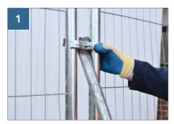
During installation, bracing can be added by removing the nut from the top coupler and connecting the support brace as shown. Tighten the nut (recommended torque 13NM) to secure the support brace.
