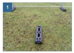
Place a rubber block mid point at the required distance in line with the first panel to be braced, as shown.
