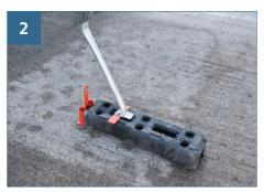
Place rubber block on ZT base and position the mini brace. Secure with bolt and plate, ensuring the mini brace is secured above the plate as shown. Unlike other installations, an additional coupler is required for use with the mini brace.
