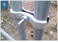
Place the next panel in position and connect to the first panel using two couplers as shown.
