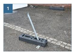
Short braces should be added at the beginning of the installation by inserting the brace through the back rectangular hole of the block, as shown.
