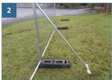
Connect the support brace as shown and tighten the nut (recommended torque 13NM) to secure the support brace, ensuring the plate is flat on the ground.
