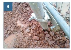
Offer the first panel up to the first tubes and connect the bottom BK clamps in place, as shown and secure bottom of panel by tightening bolts (recommended torque 7NM—5lb/ft).
