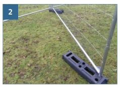
Insert a mesh panel into the round hole farthest away from the fence line as shown.
