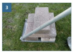
Add ballast to the loading tray and repeat along the fence line until the installation is complete.
