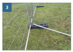
Insert the other end of the panel into the rectangular hole closest to the fence line as shown.
