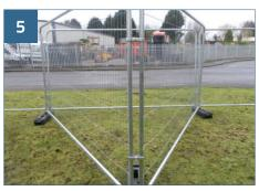
Connect both panels together us-ing two couplers as shown and tighten (recommended torque 13NM).
