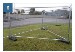
Connect both panels to the fence line using the same method as in step 5, as shown. Repeat at required intervals along the fence line until the installation is complete.
