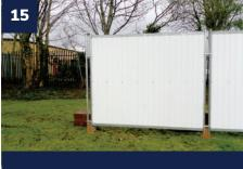
Insert a dummy tube at the end point to allow the last panel to be braced.
