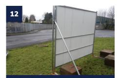
Attach the support brace onto the coupler bolt as shown and secure with nut and tighten (recommended torque 13NM or 9.5lb/ft).
