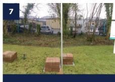
Place a dummy tube into the end hole of the first ZT base.
