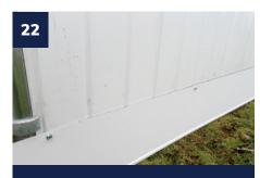
Place the first ground skirt at the start of the fence line and secure in place using two Tek screws as shown, one at the outer edge and one halfway along the skirt, ensuring they are tight.
