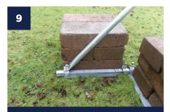
Place support brace on fourth bolt hole and re-insert and tighten bolt (recommended torque 15NM or 11lb/ft).
