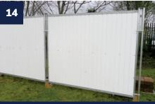
Continue to erect hoarding in the same way until installation is complete. Ensure all connections are tightened to the recommended torque settings prior to inserting the next panel.
