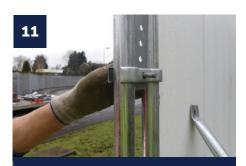
Insert the brace lock into the top tubes. Place the bolt through the coupler half and brace lock and also the second coupler half.
