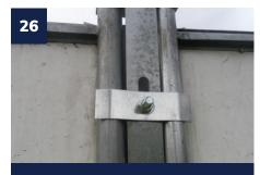
Insert the bolt through the top hole form the outside of the hoarding line through the brace lock slot and attach the backing plate on the inside of the hoarding line. Attach nut and tighten to secure the privacy infill in place (recommended torque 7NM or 5lb/ft).
