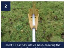
bar is touching the upright of the base as shown, and tighten bolt (recommended torque) 15NM or 11lb/ft).
