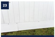
Place the next skirt in position so that it reaches halfway across the space between the panels and secure one end. This will leave an overlap in the centre of the panel, which is to be secured using the remaining screws as shown.
