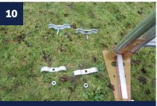
Disassemble 2 couplers as shown, and place two halves and the bolts on the outside of the fence line, the other halves and nuts on the inside of the fence line.
