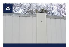
Place the infill in position covering the gap and level with the top of the panels.
