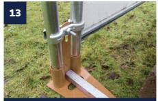
Insert the second coupler bolt through the half of the coupler and the upright of the ZT base, replace other half and nut and tighten (recommended torque 13NM or 9.5lb/ft).
