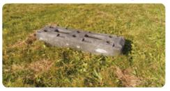
Place the first rubber block at the proposed starting point of the fence line.
