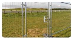
The latch pole should be placed in the next block and connected to the next panel in the fence line, ensuring the catch is lined up with the latch of the gate.
